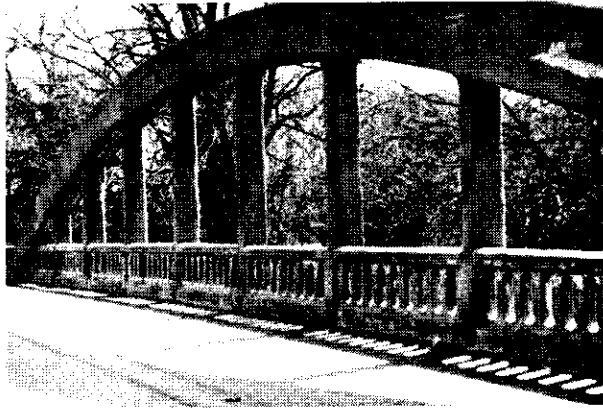
Rainbow Arch Bridge 1918 110' Single Span
