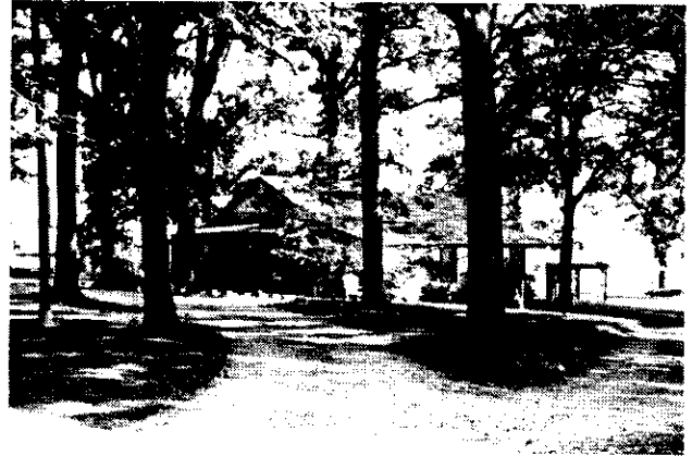
Cabin Camp Office
